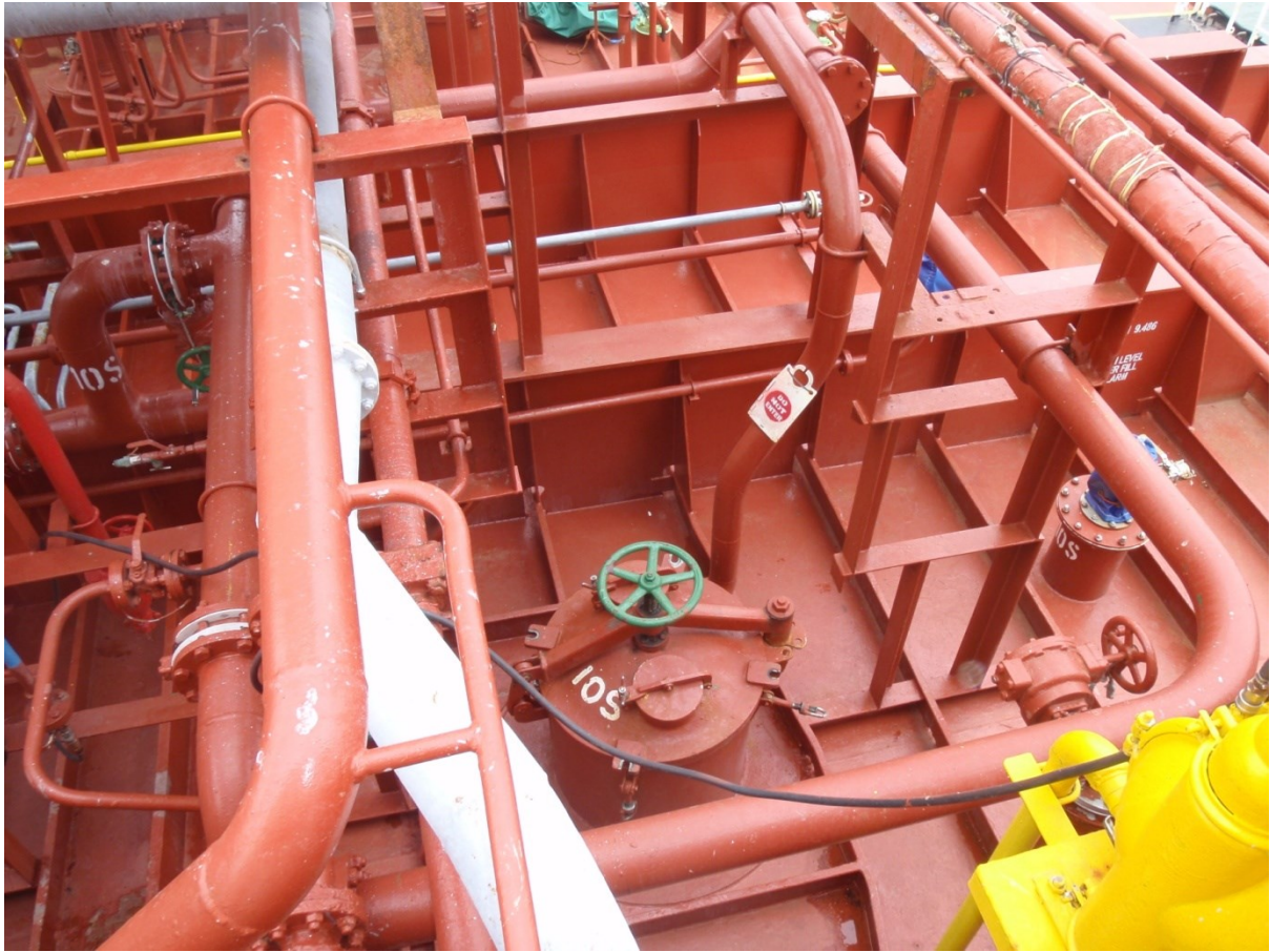
Area around the tank entrance
