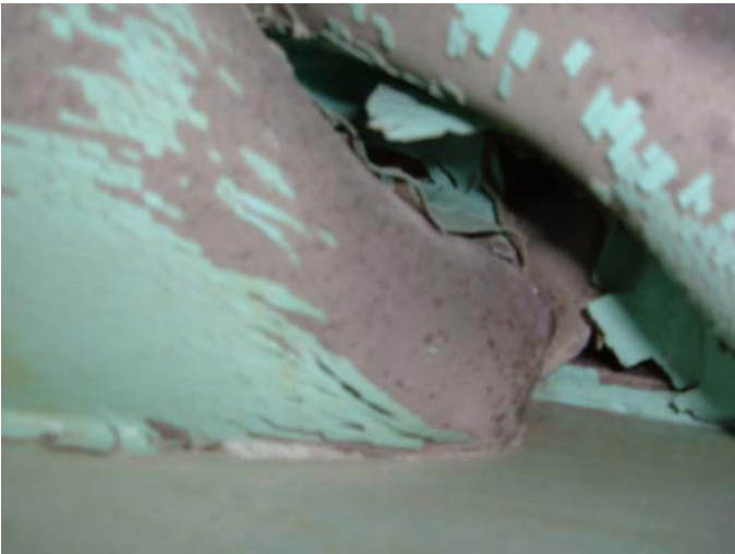
Fig 4: Damage in forepeak tank
