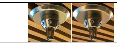
Figure 15: HI-FOG 1900 installed with (left) & without (right) a spacer
