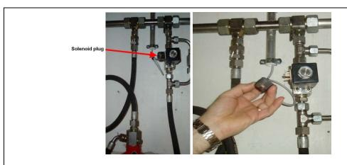
Figure 06: Disconnecting the solenoid plug from a Bürkert valve
