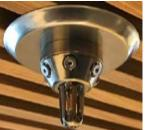
Figure 15: HI-FOG 1900 installed with (left) & without (right) a Spacer plate
