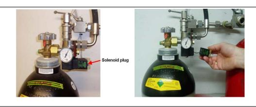
Figure 07 : Disconnecting the solenoid plug from a release valve
